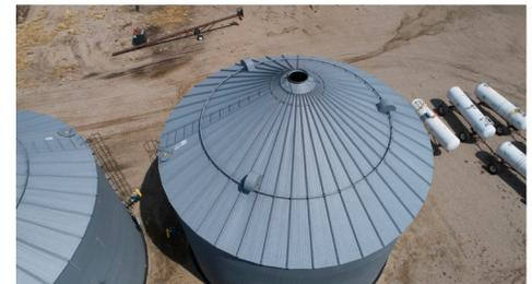
**BIN 7:** 25,000± bu. Butler bin, Y design floor aeration, side ladder, Butler 2143985 230V 42 amp single phase fan, Westgo loadout, no motor/head
