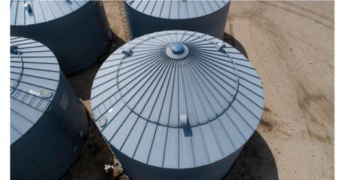
**BIN 3:** 35,000± bu. Butler bin, Y design floor aeration, side ladder, Butler 443985 230V 42 amp single phase fan, Rapat bin system powerhead loadout auger, 7.5 hp. Baldor motor, electrical panel w/(1) 110V & (2) 240V outlets
