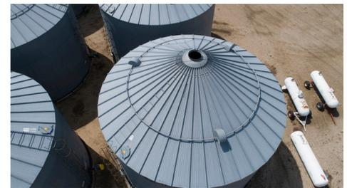
**BIN 4:** 35,000± bu. Butler bin, Y design floor aeration, side ladder, Butler 443985 230V 42 amp single phase fan, no loadout head/motor
